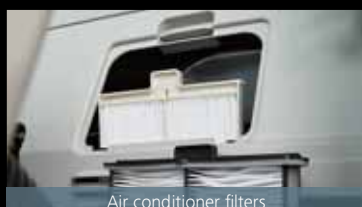
Air conditioner filters
